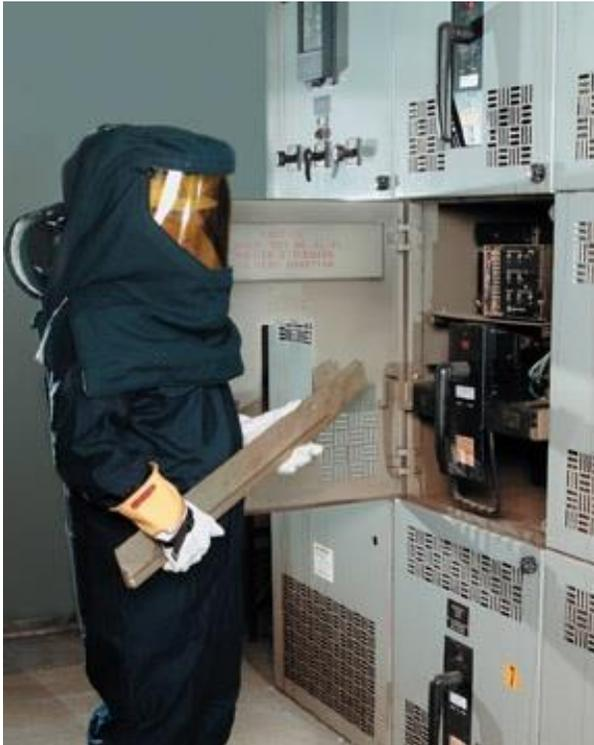
In addition to proper maintenance, increasing worker distance from electrical equipment reduces worker exposure to arc flash energy.
